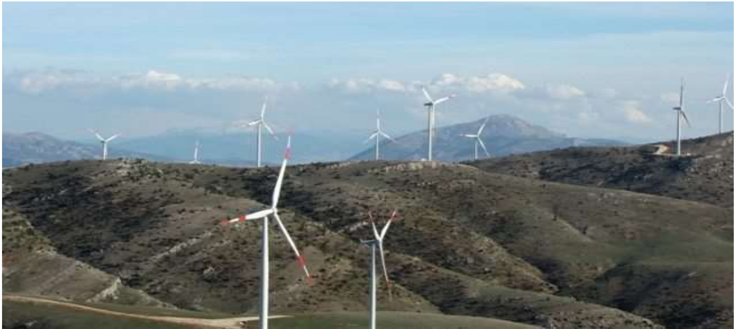
KARAGÖNLER WIND ENERGY SYSTEMS 10 MWE 2018 HATAY/Turkey
